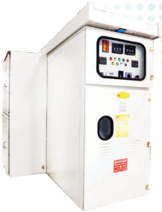
22kV VCB OUTDOOR PANEL
