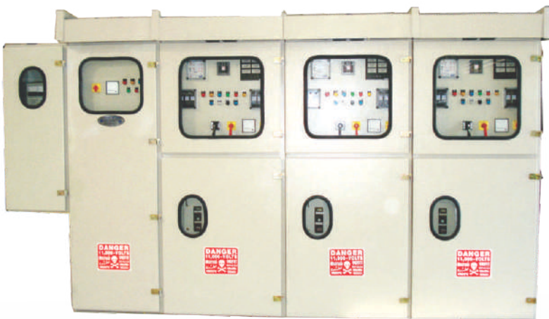
11kV OUTDOOR VCB LINE UP PANEL WITH METERING
