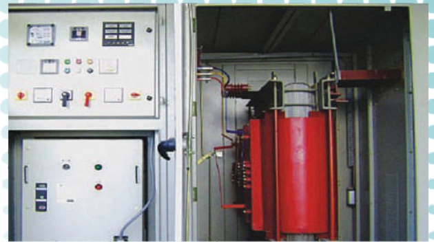
11 KV, VCB PANEL WITH TRANSFORMER
