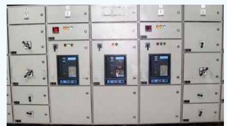
LT Main Distribution Board
