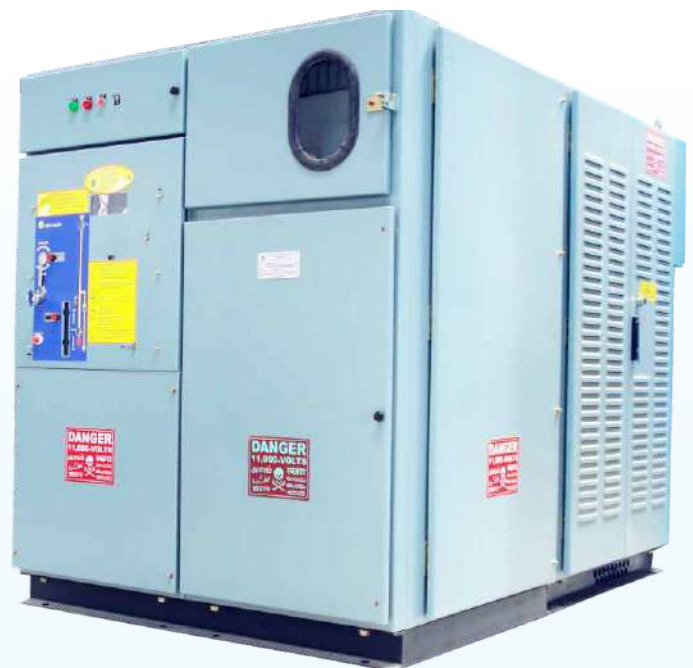
11KV 315KVA INDOOR USS WITH LBS AND KSEB METERING
