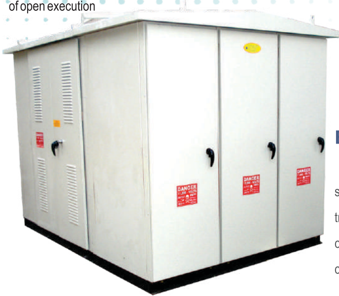
11kV, 1000kVA USS PANEL WITH RMU-OUTDOOR WITH OLTC
