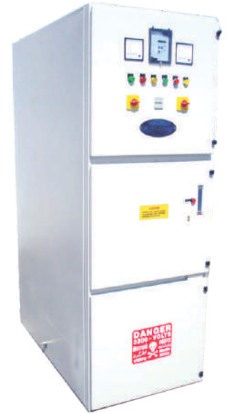
7.2kV INDOOR VACUUM CONTACTOR PANEL
